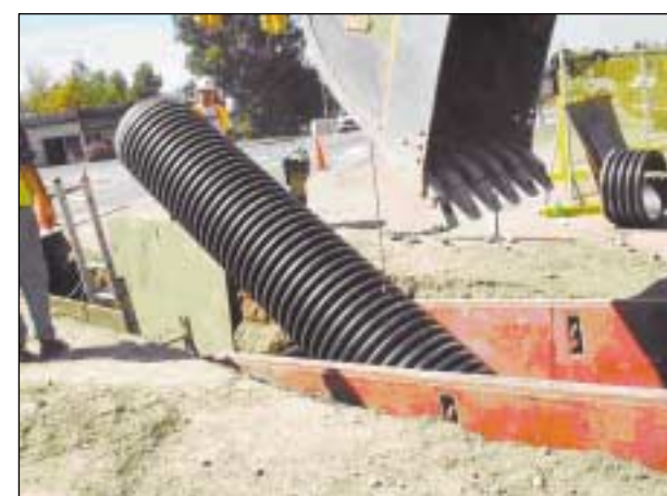
Contractor installing 30-inch storm drain on 164th Avenue SE
