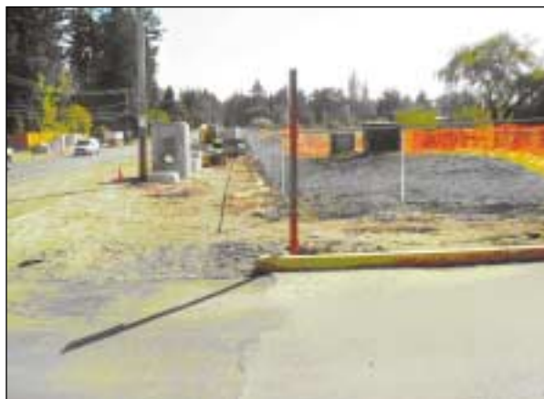
Storm drainage structures ready for installation on SE 256th Street
