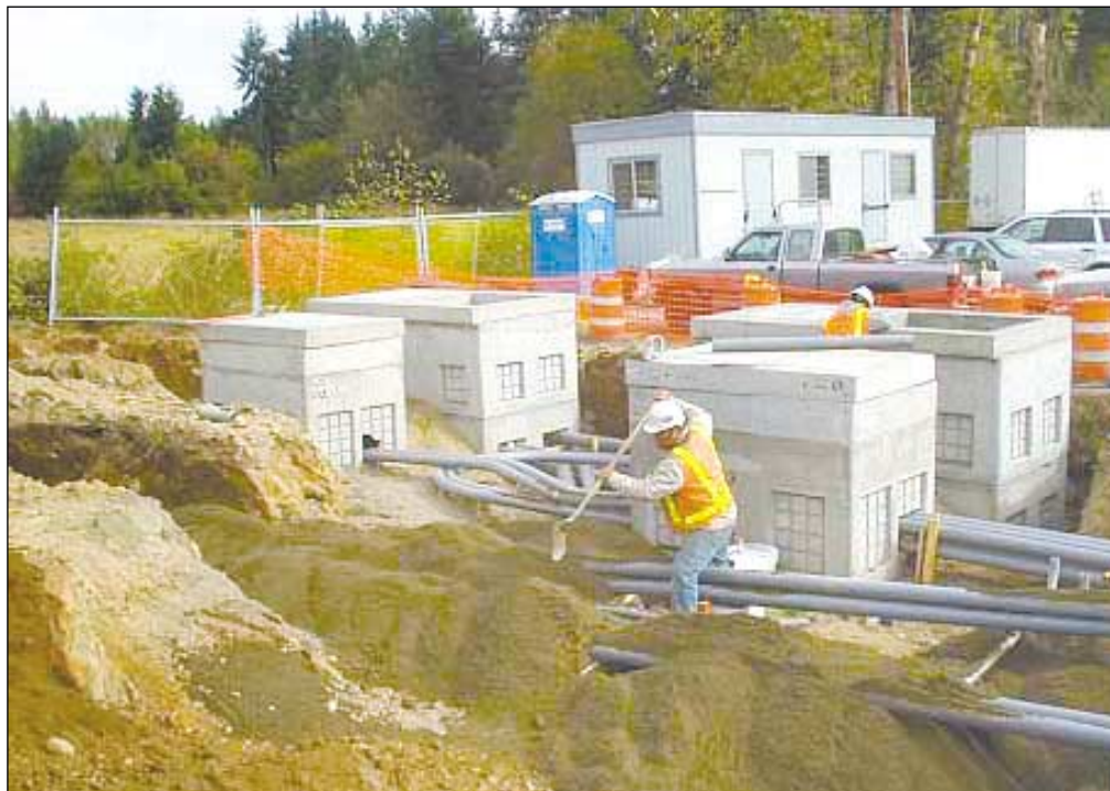
Contractor installing utility vaults and back-filling conduits with sand.
