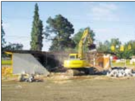
Demolition of Three French Hens
