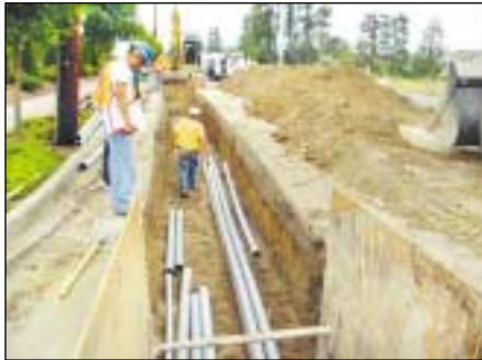
Excavation and installation of joint utilities trench on SE 256th Street
