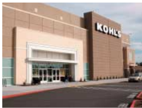
Covington Commercial Retail Center Phase II Kohl's Department Store
