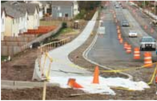
New Sidewalk on South Side of SE 256th Street
